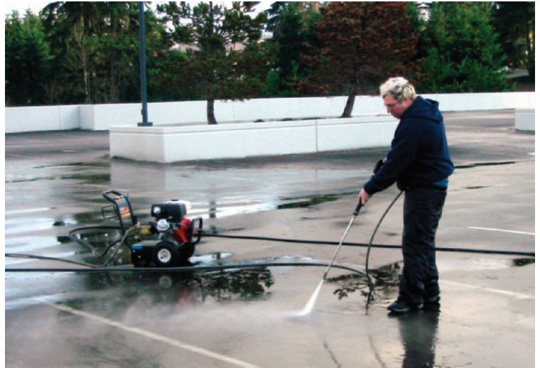
7 Pressure washing the parking deck during a rare moment when the rain stopped. Note the small width of the spray coming out of the nozzle. Because of the glare and the reflections off puddles in this image, it's hard to see where the ground has been washed and where it hasn't.
